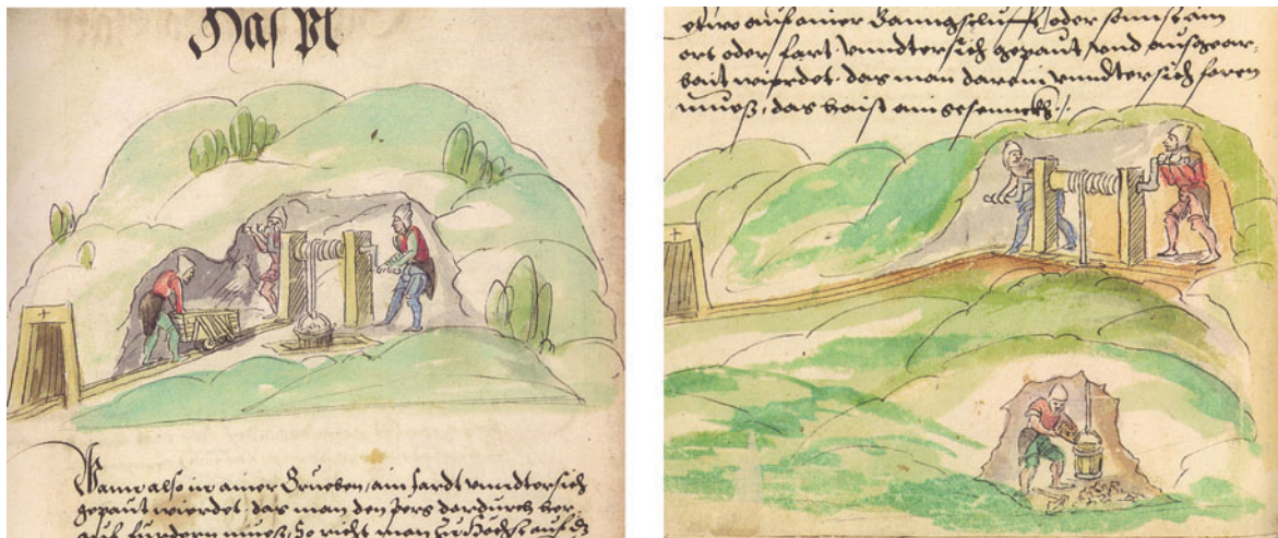
Figure 3. Winches in the draft version of the Schwazer Bergbuch (Bochum, Deutsches Bergbaumuseum, Codex Sig. 3313, pp. 48f.).
