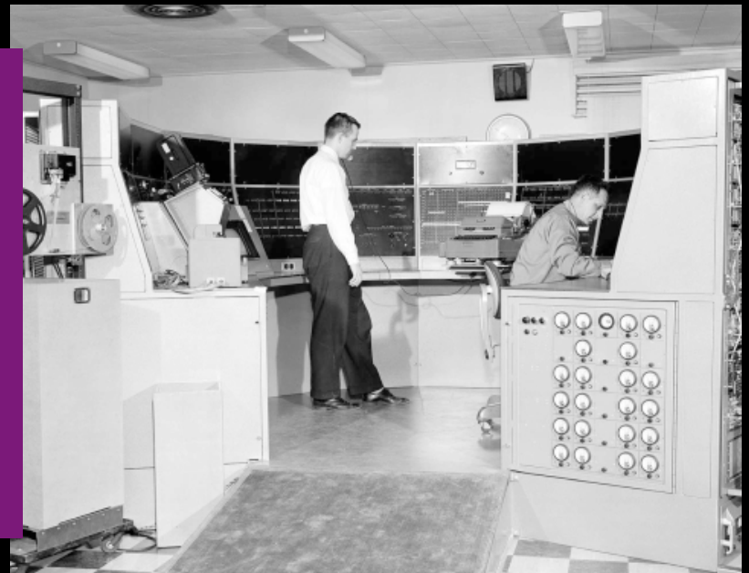
Millstone control room
